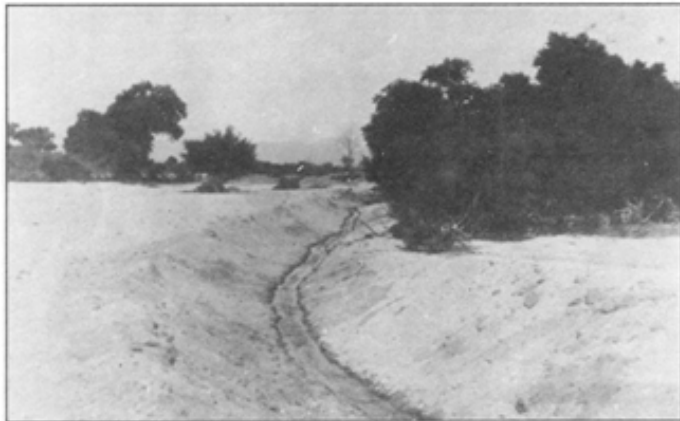
The Allison brothers' West Side Canal was built in the early 1890s to revive irrigated agriculture after the river became entrenched (photo 110. 4250 courtesy of the Arizona Historical Society).
